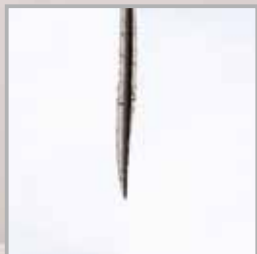
CRACKS AND TEARS CAN RETURN WITHIN DAYS
