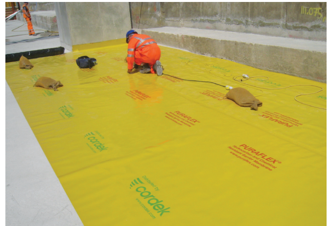
Membrane being installed
